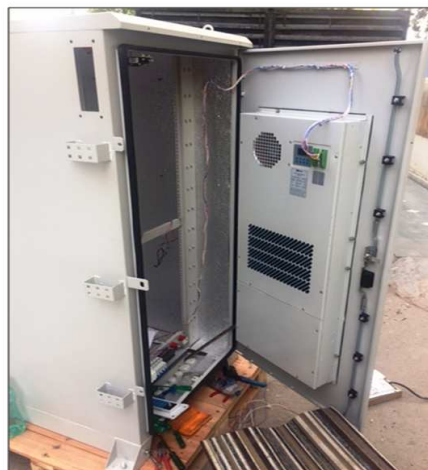
Hybrid 24U HRC with Aircon 1500W+HEX 150W/K for Heat Load 800W @ L27/L47 & Aircon 2000W+HEX 150W/K for Heat Load 1000W @ L27/L47
