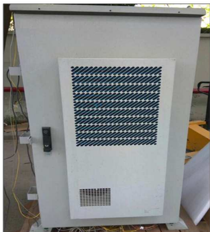
Hybrid 24U HRC with Aircon 1500W+HEX 150W/K for Heat Load 800W @ L27/L47 & Aircon 2000W+HEX 150W/K for Heat Load 1000W @ L27/L47
