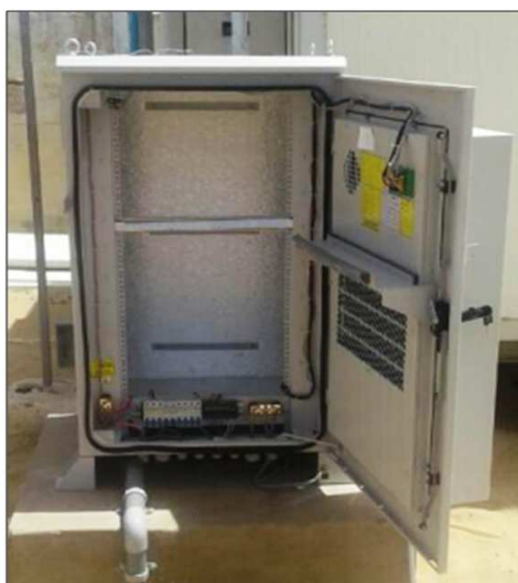
Hybrid 16U HRC with Aircon 800W+HEX 80W/K for Heat Load 500W @ L27/L47
